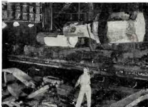
Cuts Steel Like Butter! This modern flame-cutting equipment, in use at U.S. Steel Supply Division warehouses, can follow the most complicated patterns accurately and turn out finished shapes of steel exactly as wanted. Many fabricators of steel products buy their steel from U.S. Steel Supply, and have it cut to shape before it is delivered to them.
